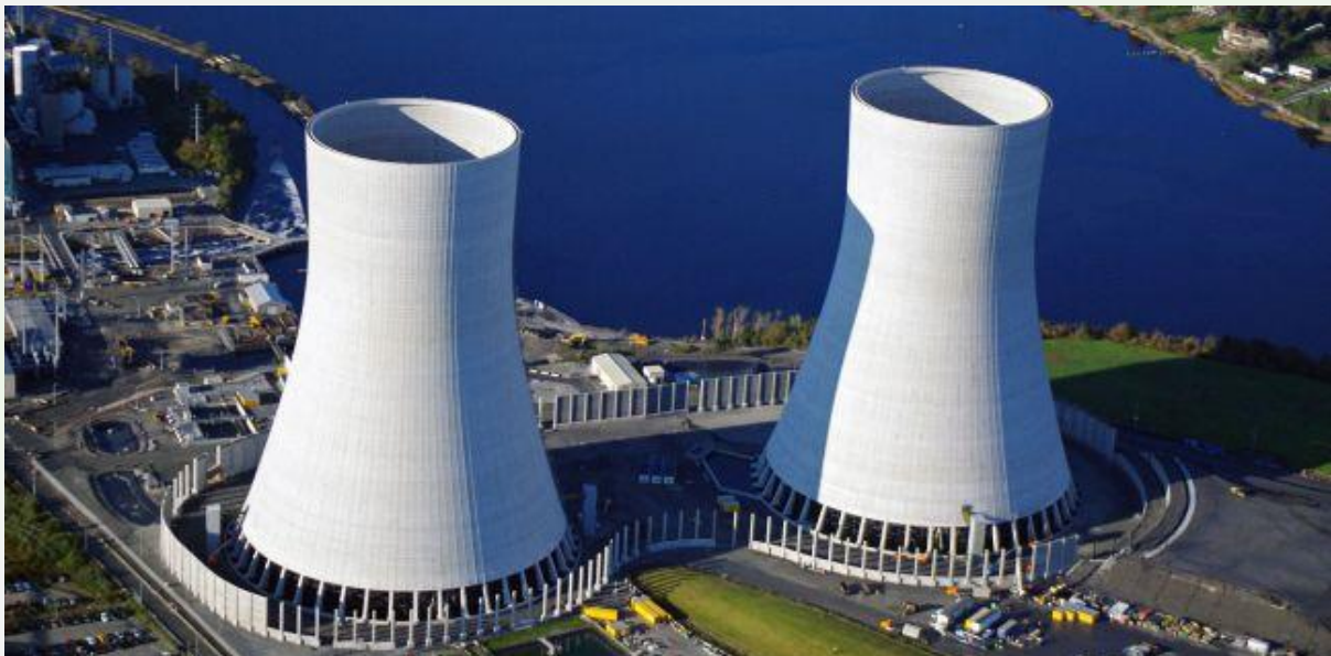
Fig. 2: Cooling Towers in Electric Industries
