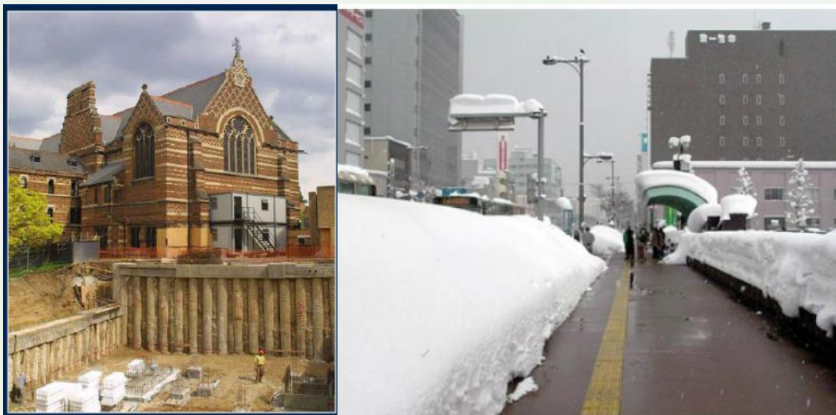
Fig. 1: Implementation of Energy Piles in: Left) Keble College, UK. and, Right) a Walk Road in Japan
